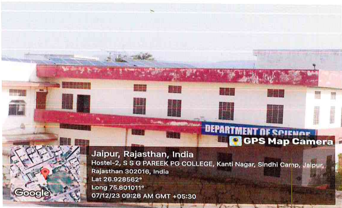
Solar Panel on Science Block
