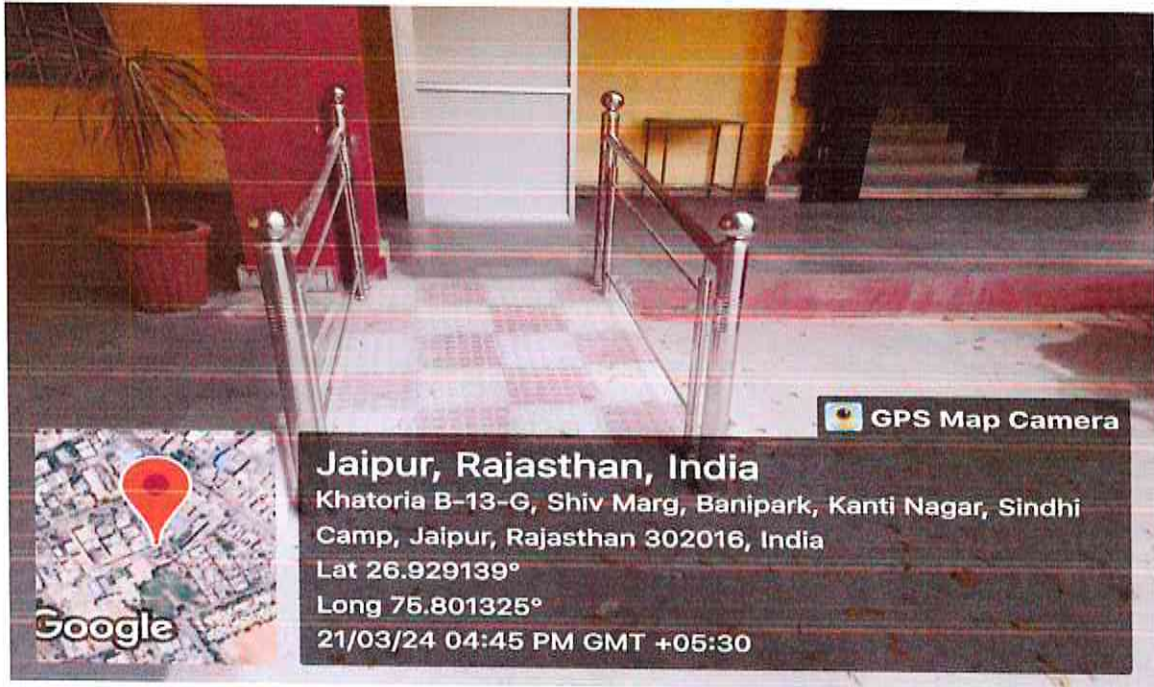
Ramp in Science Block
